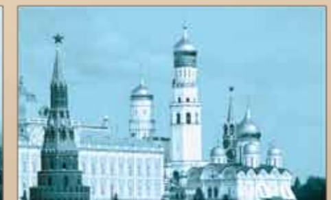
THE KREMLIN Trane landmark building since 1991
